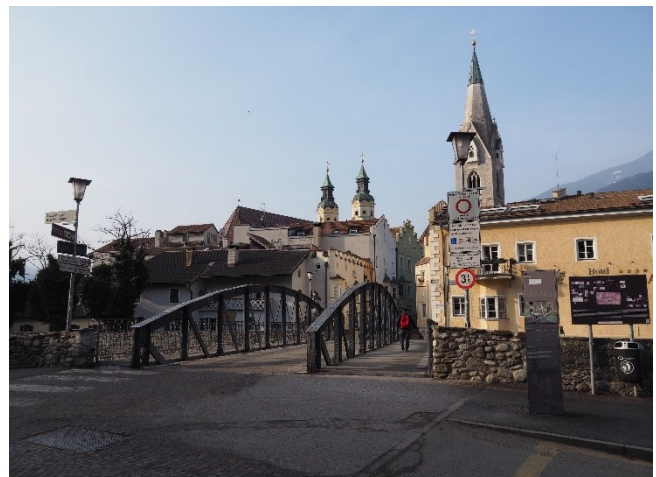
Adlerbrücke – Blick Richtung Westen Ponte Aquila – Vista verso ovest
